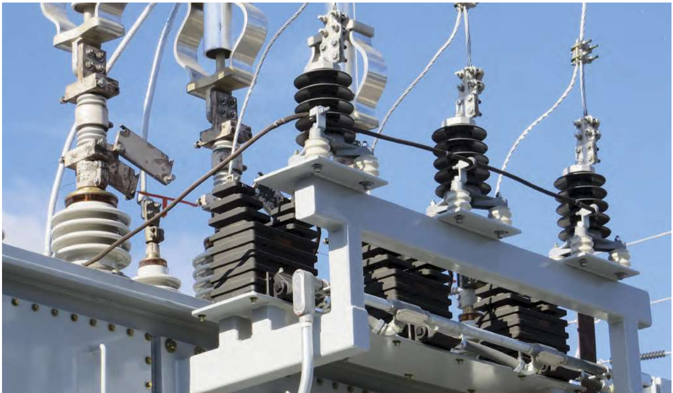
Improvement in production technology is key to reduction in energy consumption.
