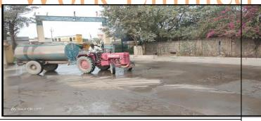
Water Sprinkling through Water Tankers
