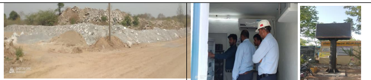
A Visual of Garland drain around the dump yard
