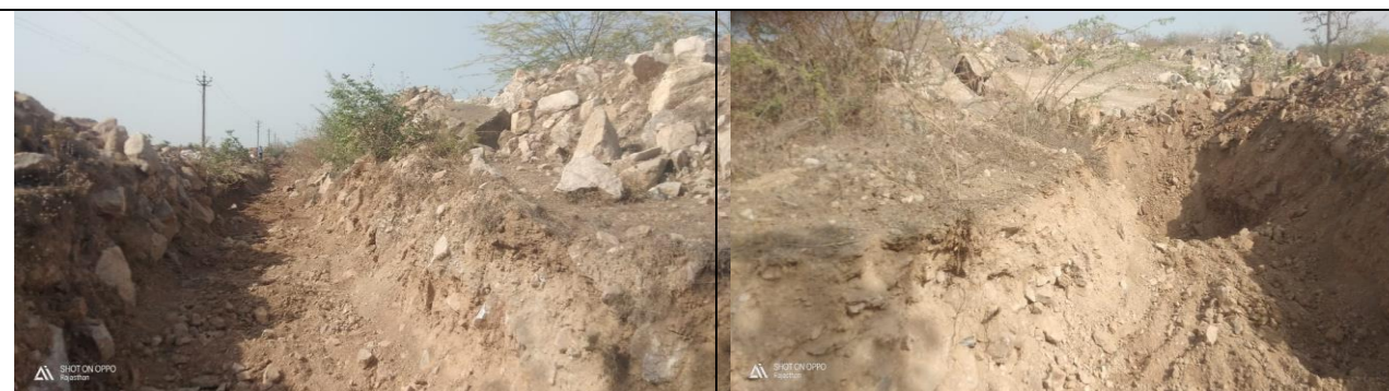
A Visual of Garland drain around the dumps to arrest silt and sediment flows.
