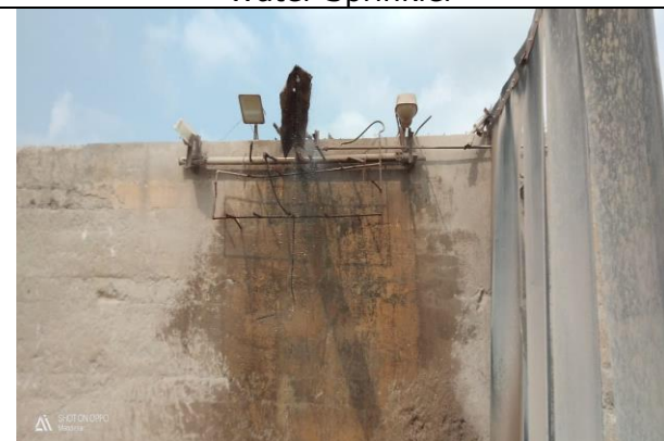
Water Sprinkling system at Crusher hopper
