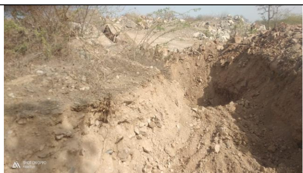
A Visual of Garland drain around the dumps to arrest silt and sediment flows.
