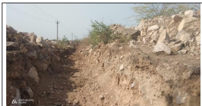
A Visual of Garland drain around the dumps to arrest silt and sediment flows.
